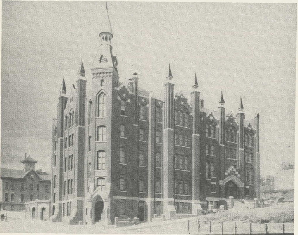
Cooper Medical College. Original building with addition including Lane Hall, ca. 1892.
